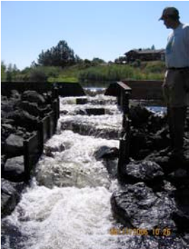
Photo of fish ladder in completed irrigation diversion project
